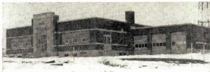
WTAG's transmitter building.
